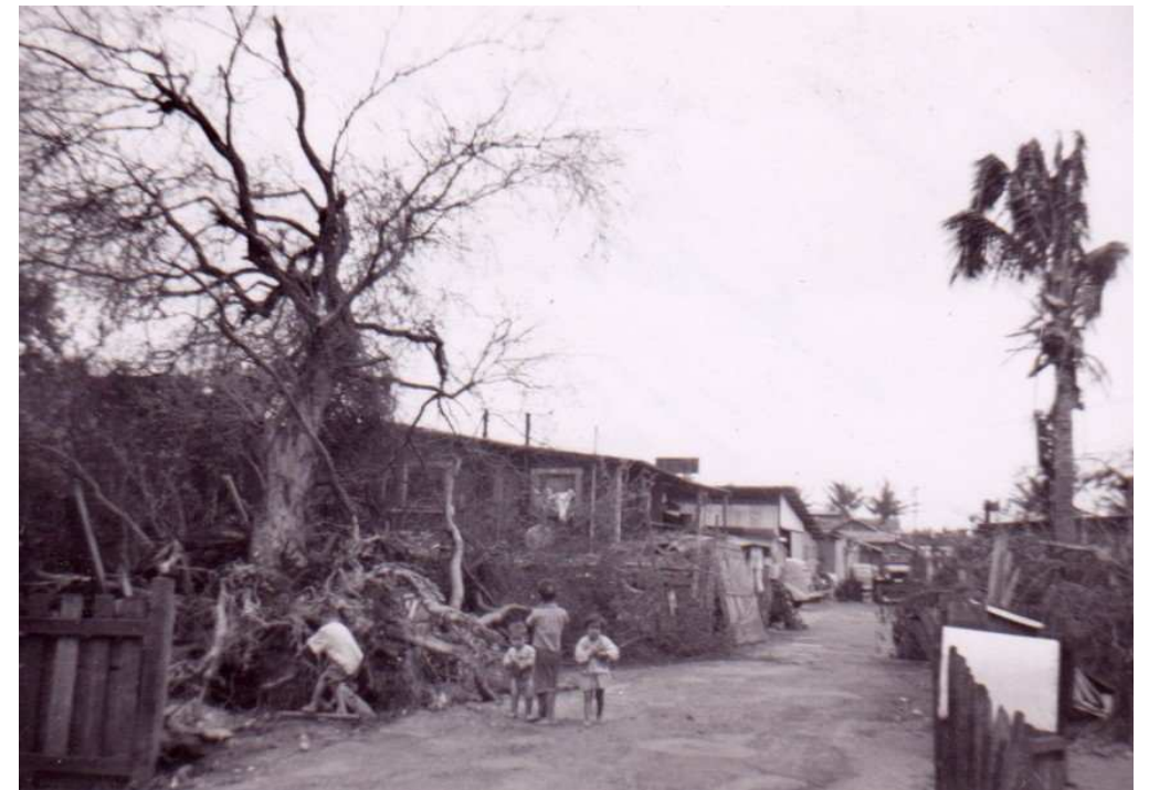
Above: Damage on Lana Lane from wind storm.
